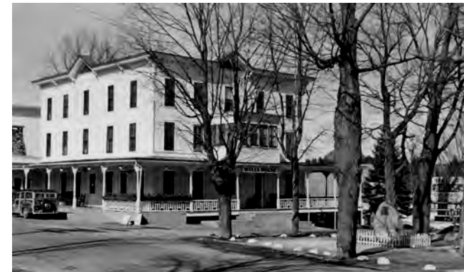
Wells House in Pottersville
