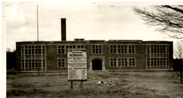
Former Chestertown Central School Under Construction - 1935
